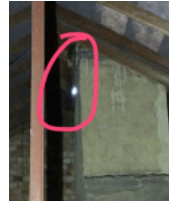
The Willows: Examples of defects Top: ceiling damaged by roofer Visible gap in chimney flashing Vent pipe replaced where penetrating roof but existing hole not repaired Centre: poor workmanship: sundry leaks, incomplete lining to roof Bottom: leaking replacement downpipes, possibly undersized, and displaced leak guard Unfixed and poorly installed soffit
