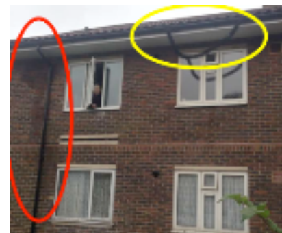
The Willows: Examples of defects Top: ceiling damaged by roofer Visible gap in chimney flashing Vent pipe replaced where penetrating roof but existing hole not repaired Centre: poor workmanship: sundry leaks, incomplete lining to roof Bottom: leaking replacement downpipes, possibly undersized, and displaced leak guard Unfixed and poorly installed soffit
